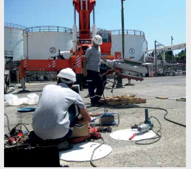
BP Mobil Shell Opet Havacılık Terminal / İstanbul, 2011
