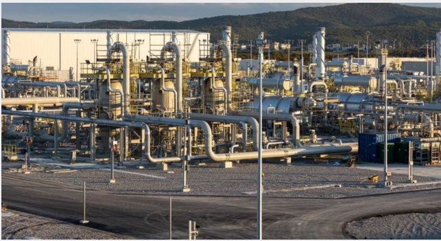
TurkStream Natural Gas Pipeline Construction Work
