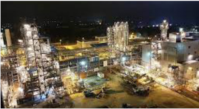
Sumqayit NTS Reconstruction Project Azerbaijan / SOCAR
