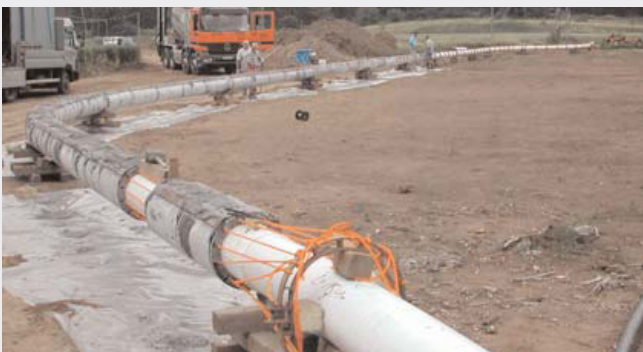
NATO Oil Pipeline Project
