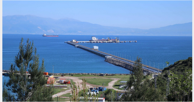
Baku - Tbilisi - Ceyhan Crude Oil Pipeline Project
