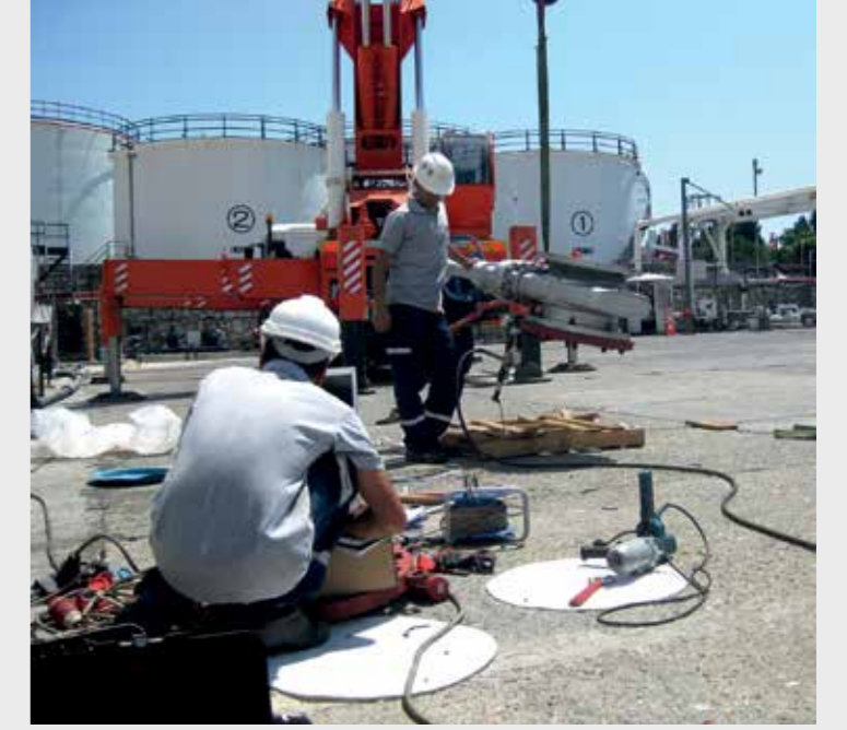
BP Mobil Shell Opet Havacılık Terminal / İstanbul, 2011
