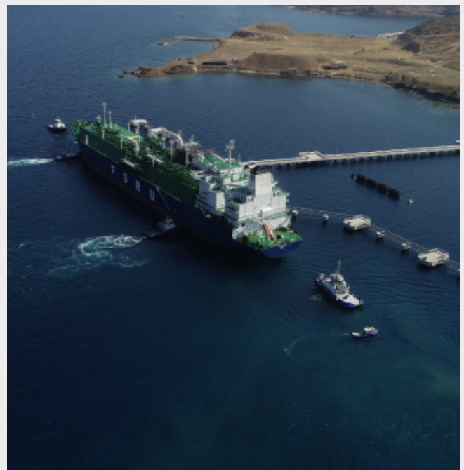
Etki LNG FSRU Terminal Regulating & Metering Station Project Turkey / Etki - Gem
